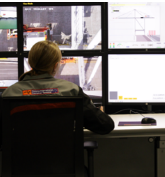
VICT's STS Automation Controller, in the office 1.2 kilometres away from ship-to-shore cranes
